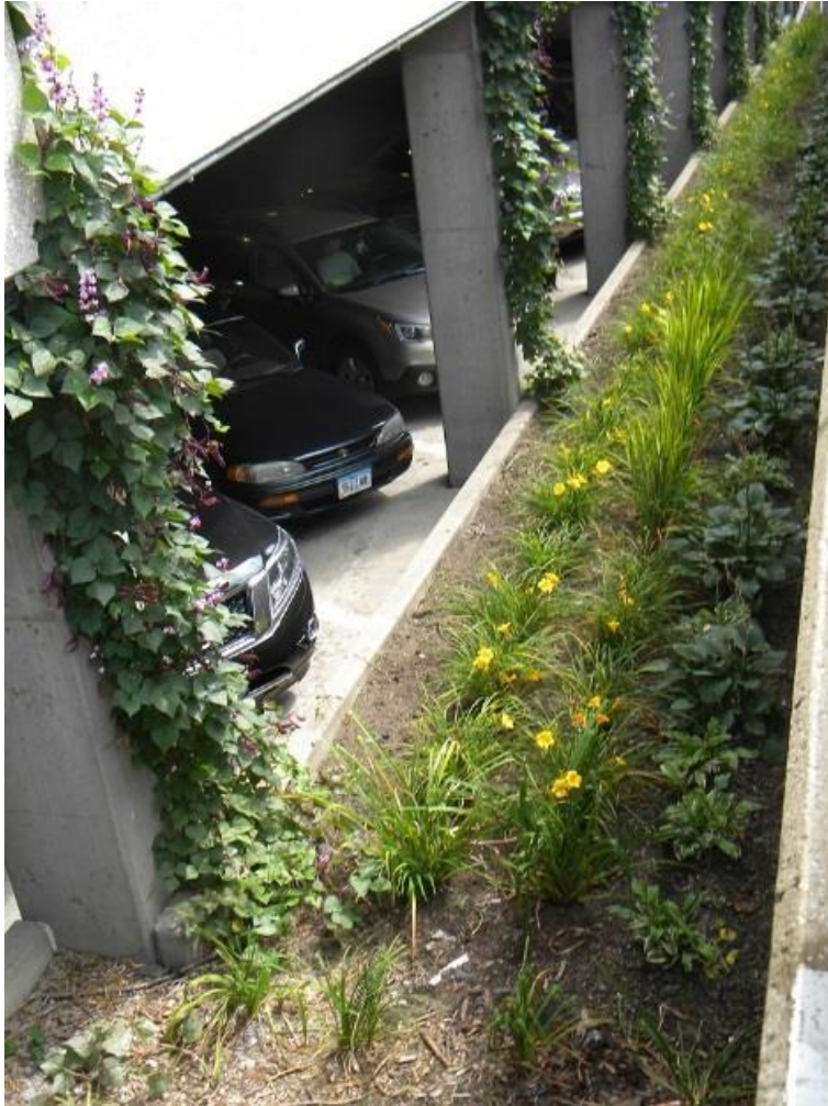
Figure 3: Close plantings will grow in; do not need mulch (Burlington St., near Sheraton)
