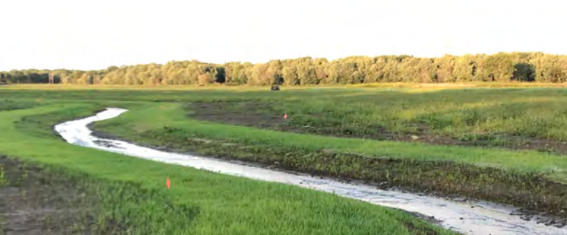
Clockwise from far left at Cedar River Crossing: A previously channelized stream was re-meandered to restore the natural hydrology; Heavy machinery from CJ Moyna restore wetlands; Volunteers help plant aquatic plants; A view of the 12,000 plants in new wetlands at CRC
